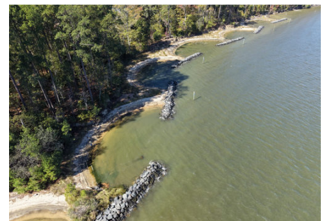
Looking north along Phase 1C
