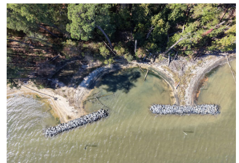
Aerial view of portion of Phase 1C
